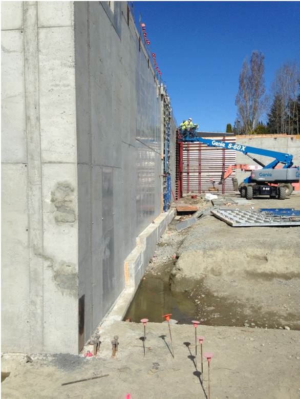
Cornerstone carpenters and concrete workers have formed and poured 3,000 Cubic Yards of Stanwood RediMix concrete
