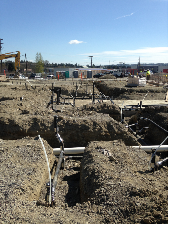
Electricians from Milne and plumbers from Ramsett have been installing underslab conduit and piping
