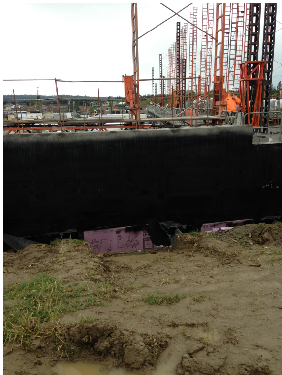
Trinity has covered 14,500 square feet with below grade waterproofing
