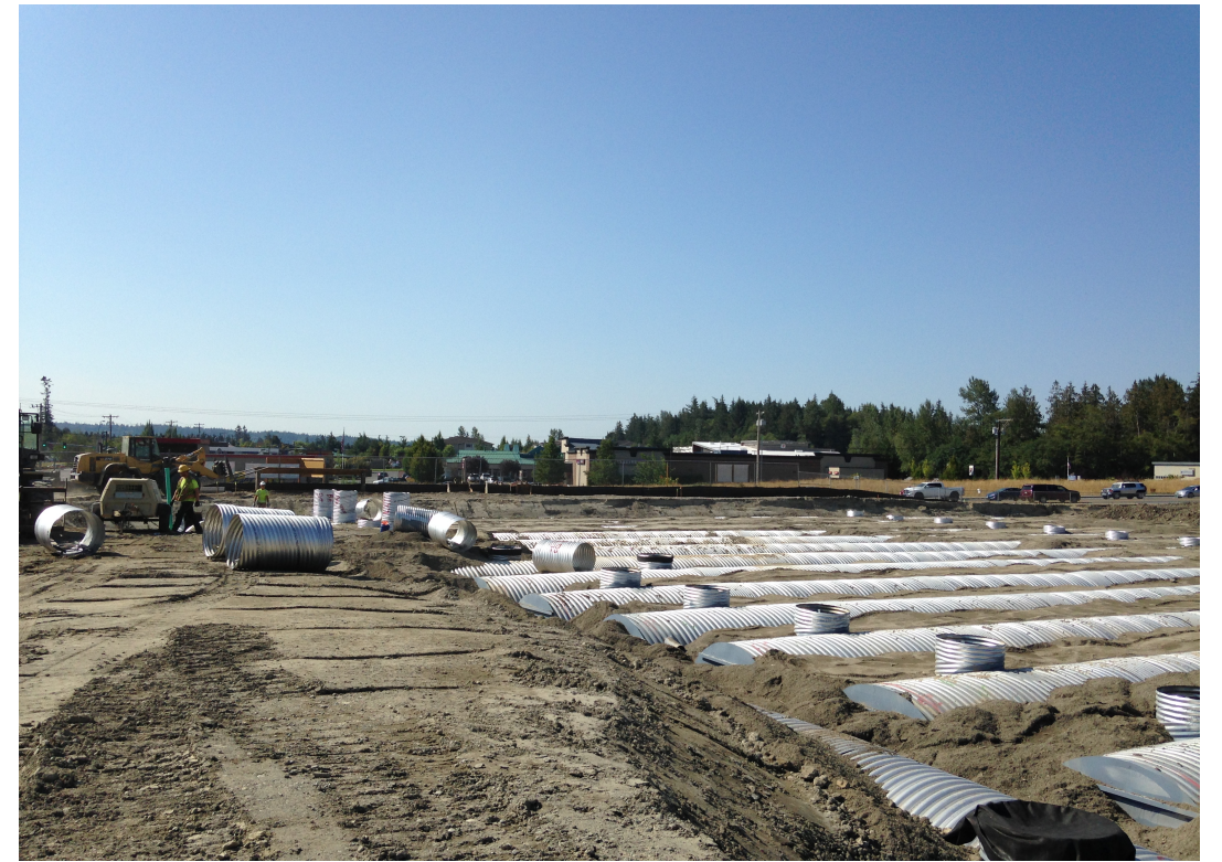
TayEx has moved 32,000 Cubic Yards of earth on site, had Lenz haul 45,000 CY, imported 95,000 Tons of structural fill, and installed 3,600 linear feet of Corrugated Metal Pipe
