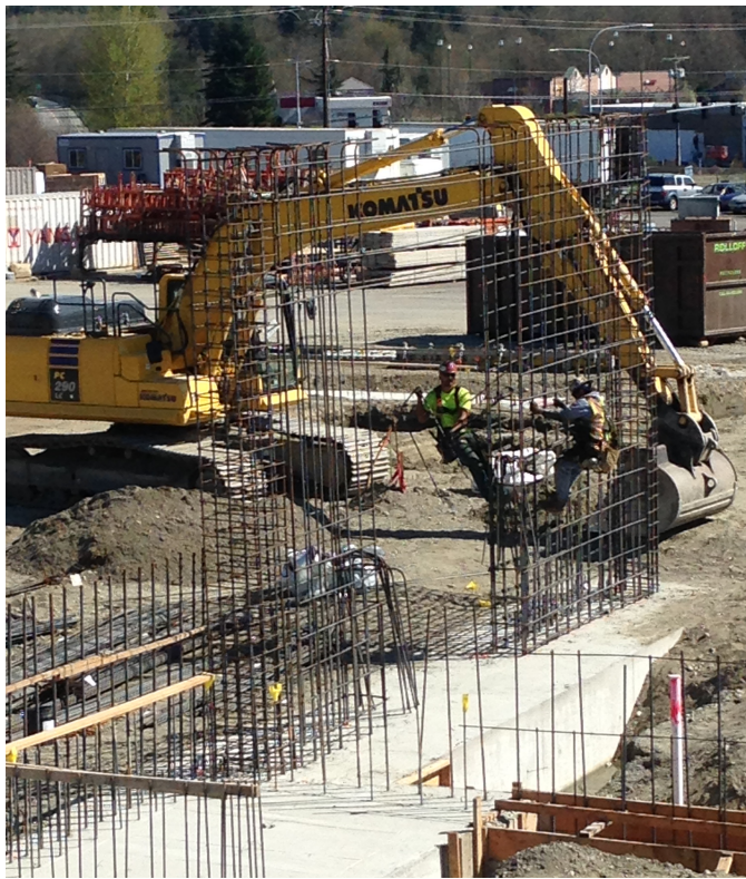
Ironworkers from Morse Steel have assembled 400 tons of rebar
