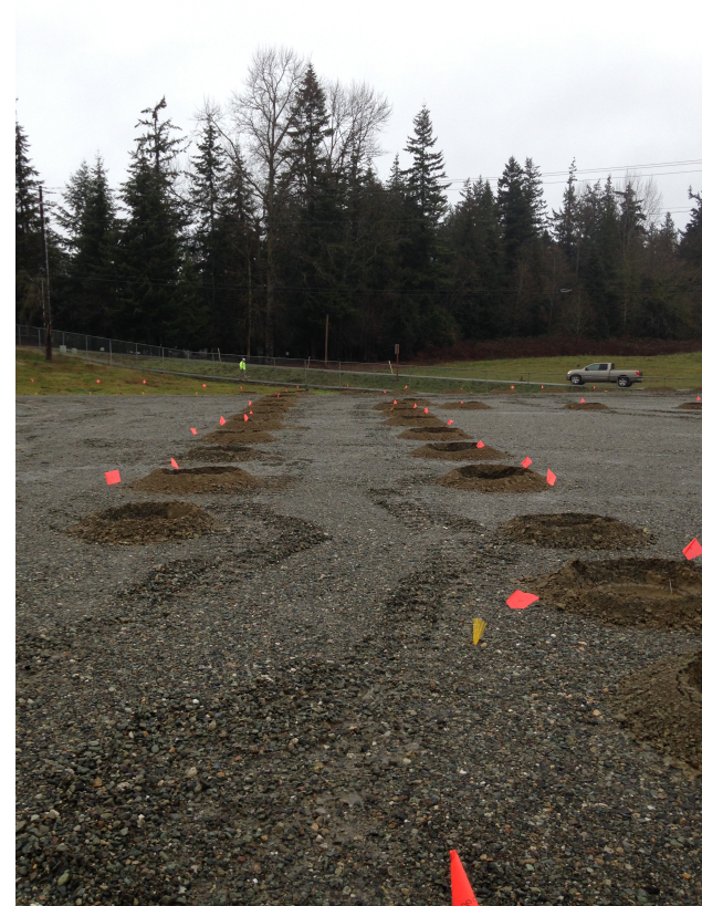
Hayward Baker installed 997 aggregate piers utilizing 4,432 tons of 1 ¼" crushed rock
