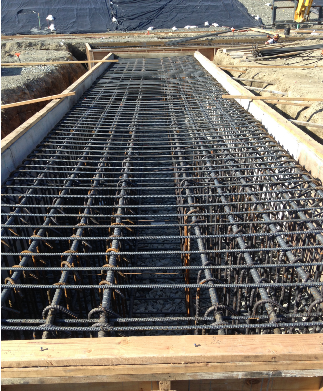
Ironworkers from Morse Steel have assembled 400 tons of rebar
