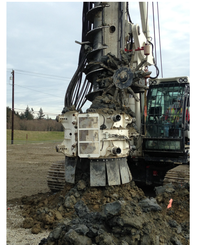
Hayward Baker installed 997 aggregate piers utilizing 4,432 tons of 1 ¼" crushed rock
