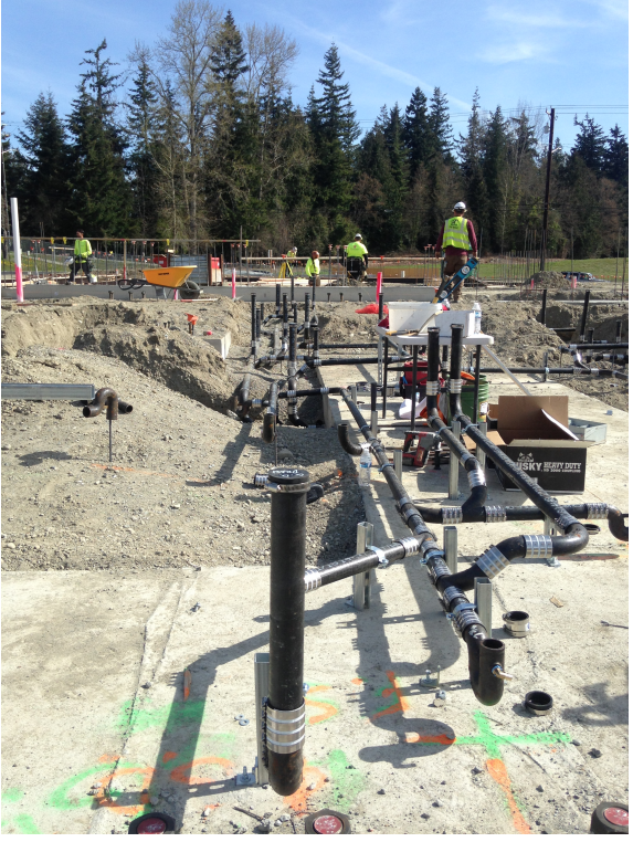
Electricians from Milne and plumbers from Ramsett have been installing underslab conduit and piping
