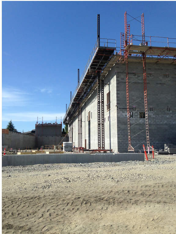
Masons from R&D have laid 18,000 CMU blocks (about 350 Tons)
