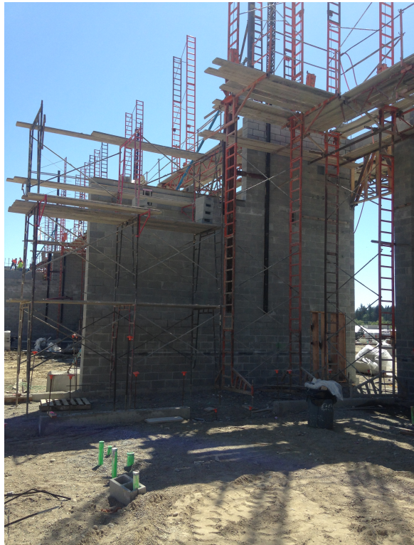
Masons from R&D have laid 18,000 CMU blocks (about 350 Tons)
