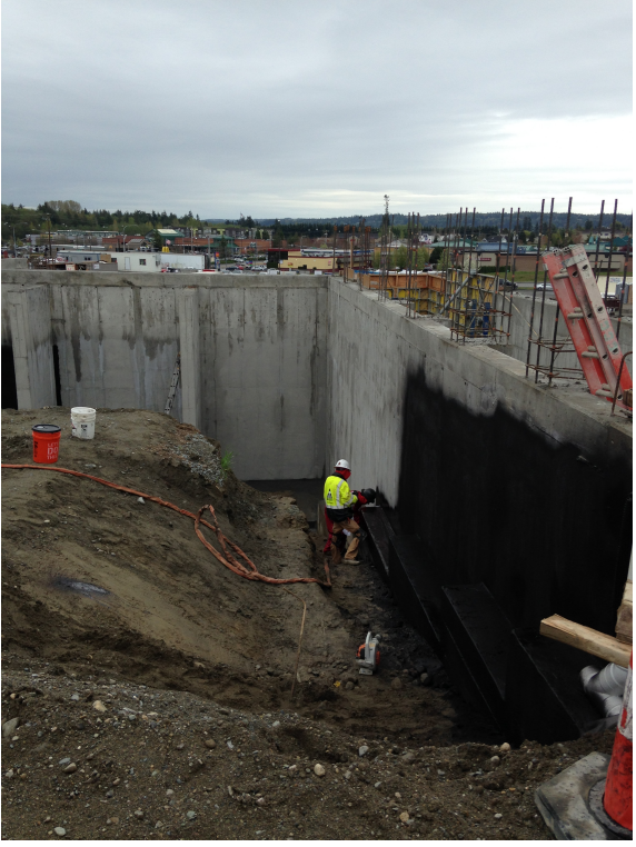
Trinity has covered 14,500 square feet with below grade waterproofing
