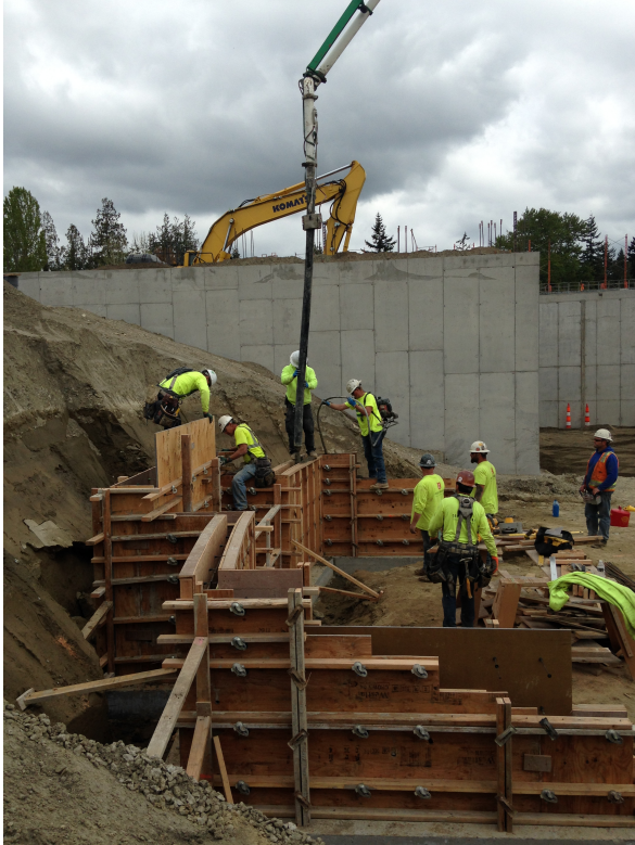
Cornerstone carpenters and concrete workers have formed and poured 3,000 Cubic Yards of Stanwood RediMix concrete
