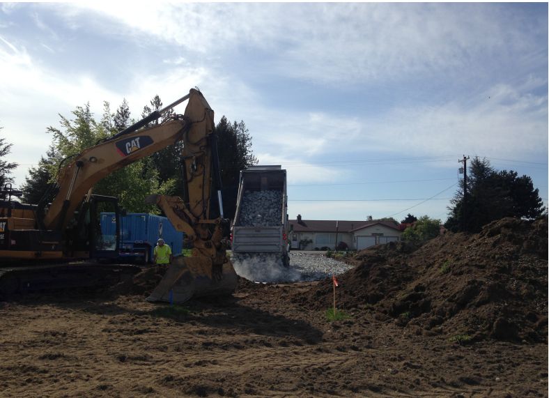
Quarry spalls being placed for the construction access drives
