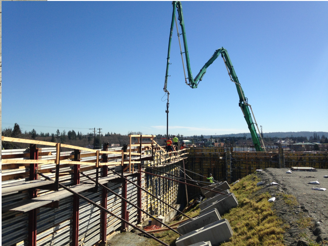
Cornerstone carpenters and concrete workers have formed and poured 3,000 Cubic Yards of Stanwood RediMix concrete
