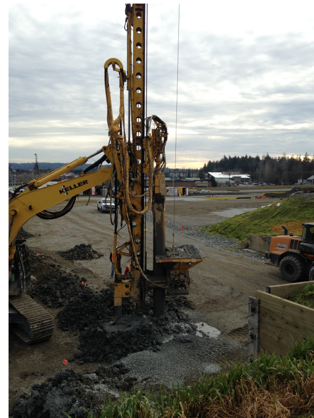
Hayward Baker installed 997 aggregate piers utilizing 4,432 tons of 1 ¼" crushed rock
