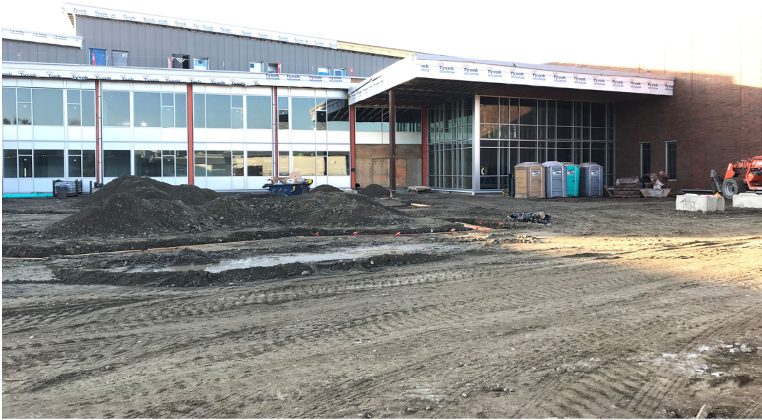
View of north elevation at student/PAC entry
