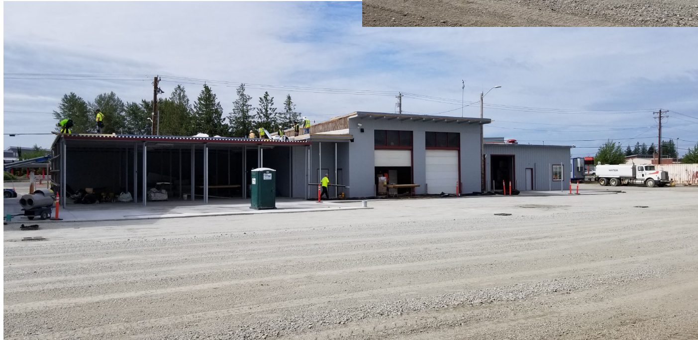
MTC Building View from the North
