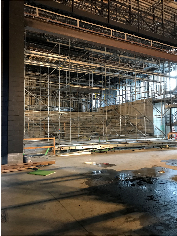
PAC scaffolding from stage
