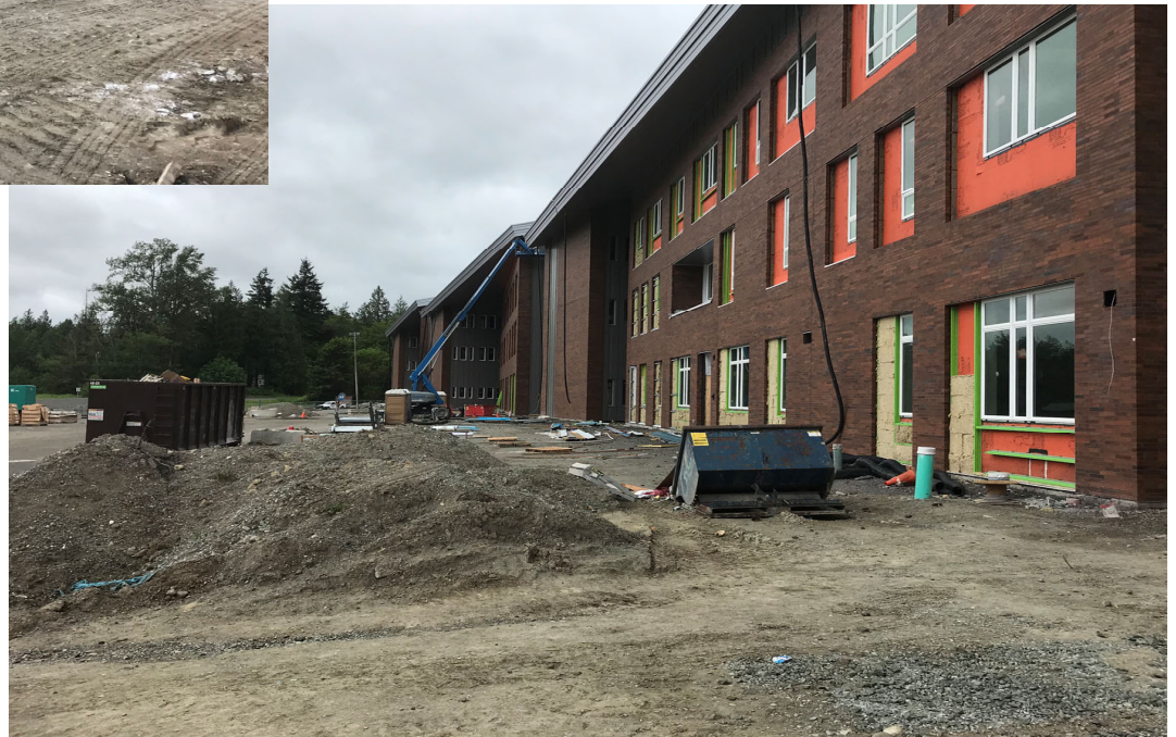
View of south elevation from Commons entry
