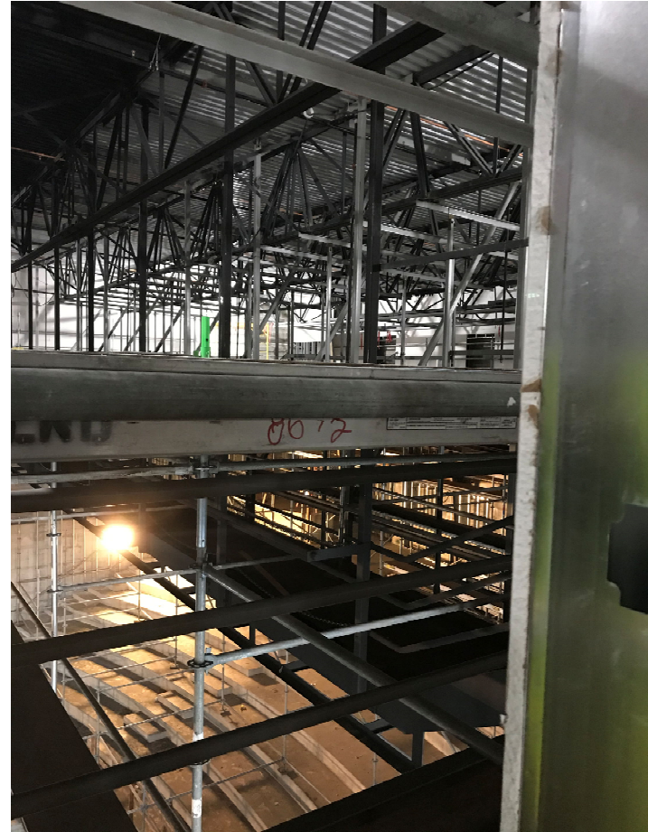
PAC scaffolding from catwalk
