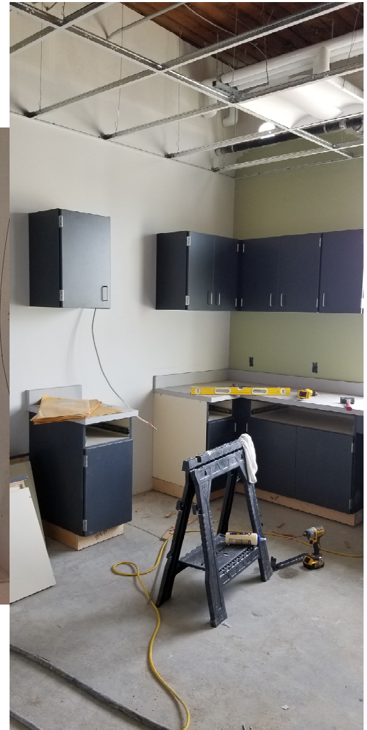
MTC Breakroom Casework
